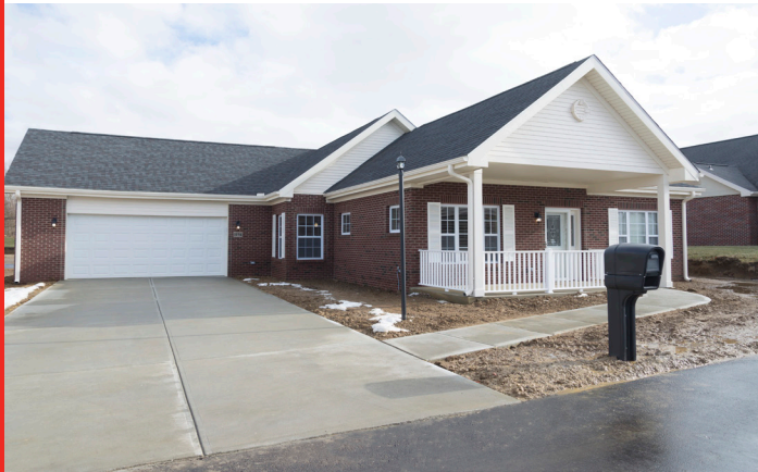
EXTERIOR ELEVATION OF COTTAGE AT LEGACY VILLAGE
