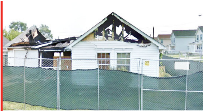
PHOTO OF EXTERIOR FIRE DAMAGE TO HOME ON DANNER AVE.
