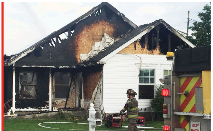
DAYTON FIRE CREWS ATTEMPT TO CONTROL THE HOUSE FIRE ON DANNER AVE.
