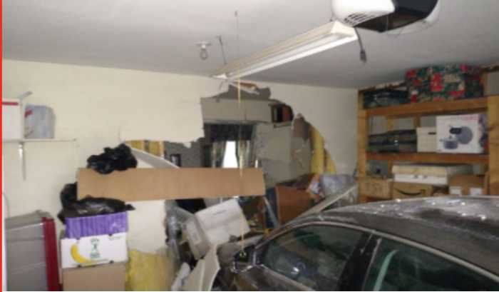
PHOTO OF DAMAGE TO THE INTERIOR GARAGE AREA -PHOTO COURTESY OF MICHAEL JASKOLKA
