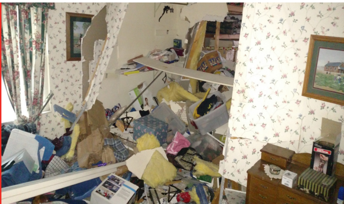
PHOTO OF INTERIOR DAMAGE AT MERRICK RESIDENCE -PHOTO COURTESY OF MICHAEL JASKOLKA
