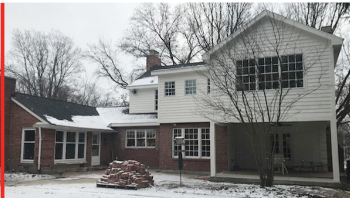
PROGRESS PHOTO OF REAR ELEVATION AT MOBLEY RESIDENCE -PHOTO COURTESY OF VICTOR ROONEY
