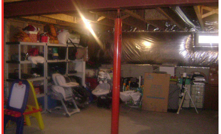
BEFORE PHOTO OF BRANNAN BASEMENT –PHOTO COURTESY OF VICTOR ROONEY
