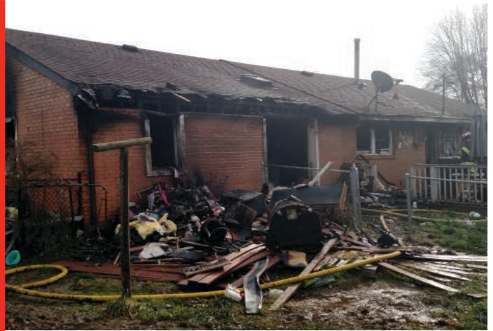
REAR ELEVATION OF WILLIAMS RESIDENCE AFTER FIRE LOSS
