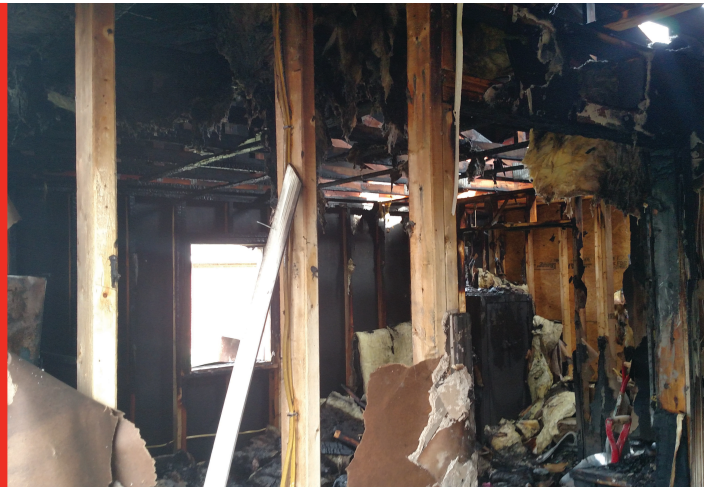
INTERIOR DAMAGE AT WILLIAMS RESIDENCE AFTER FIRE LOSS
