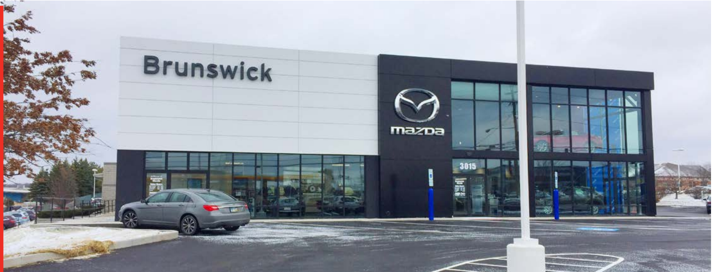
AFTER PHOTO OF BRUNSWICK MAZDA'S RENOVATED FRONT ELEVATION
