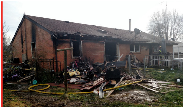
REAR ELEVATION OF WILLIAMS RESIDENCE AFTER FIRE LOSS - PHOTO COURTESY OF MICHAEL JASKOLKA
