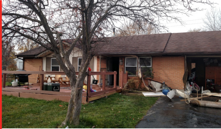
FRONT ELEVATION OF WILLIAMS RESIDENCE AFTER FIRE LOSS - PHOTO COURTESY OF MICHAEL JASKOLKA
