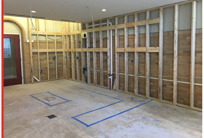
PROGRESS PHOTO OF DEMONSTRATION KITCHEN AT MIAMI VALLEY HOUSING OPPORTUNITIES - PHOTO COURTESY OF CAROLINE MORGAN
