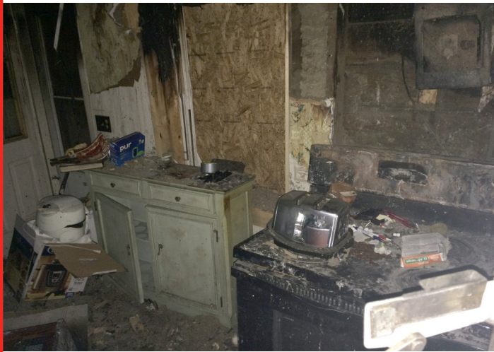
INTERIOR DAMAGE OF CURRENT RESIDENCE AFTER FIRE LOSS
