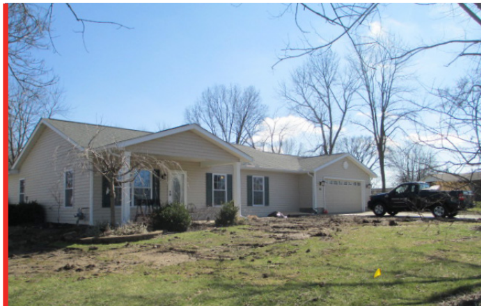
PROGRESS PHOTO OF FRONT ELEVATION AT BOWLING RESIDENCE
