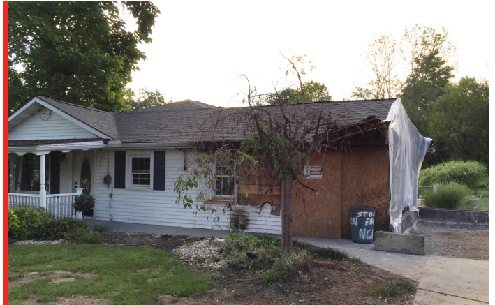
BOWLING RESIDENCE AFTER PARTIAL DEMOLITION
