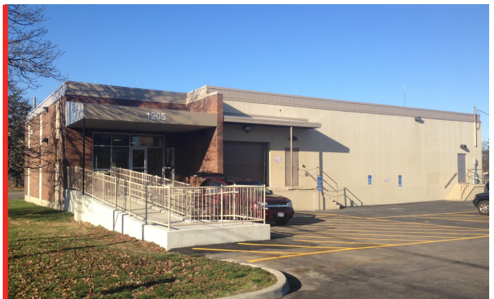
EXTERIOR PHOTO OF MONTGOMERY COUNTY ESC ANNEX AFTER RENOVATIONS
