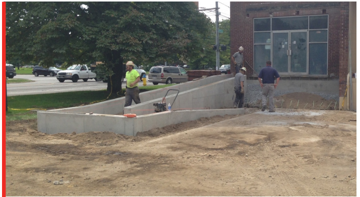
DURING PHOTO OF EXTERIOR RENOVATIONS AT MONTGOMERY COUNTY ESC
