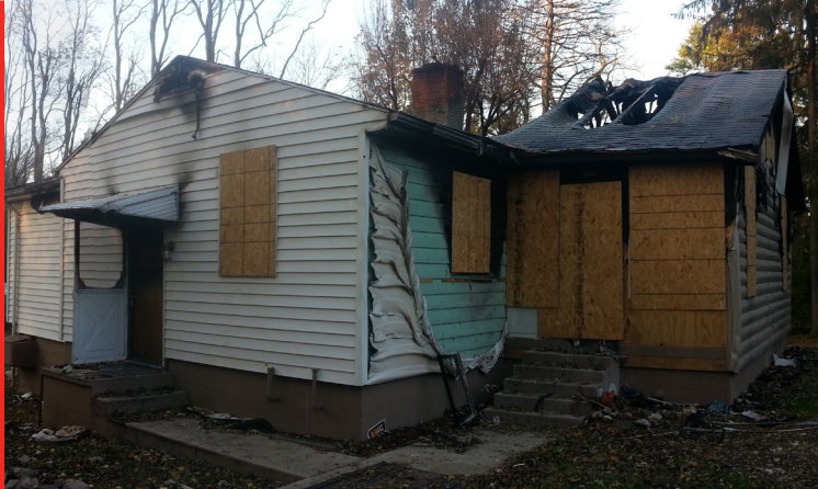
SIDE ELEVATION OF TYREE RESIDENCE AFTER FIRE LOSS - PHOTO COURTESY OF MICHAEL JASKOLKA
