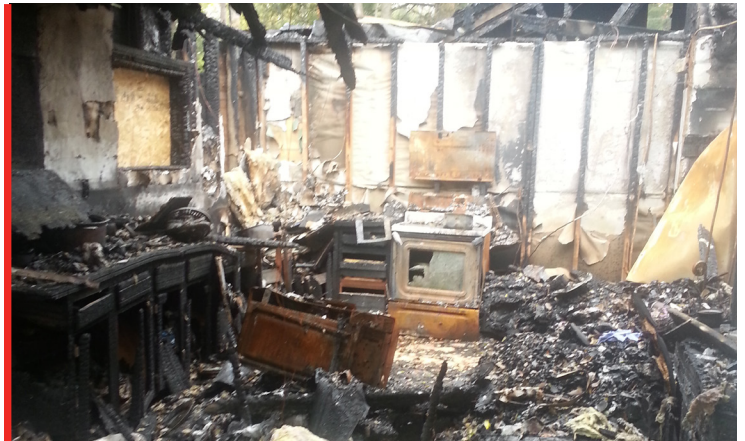
KITCHEN AT TYREE HOME AFTER FIRE LOSS - PHOTO COURTESY OF MICHAEL JASKOLKA
