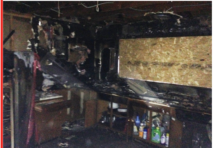
PHOTO OF FIRE DAMAGE AT REYNOLDS RESIDENCE
