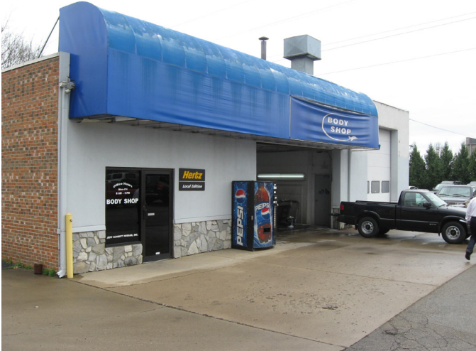
Existing Body Shop at Jeff Schmitt Nissan in Beavercreek, Ohio.
