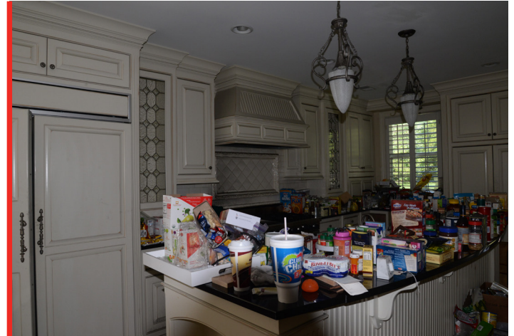
SMOKE-DAMAGED KITCHEN IN OAKWOOD HOME
