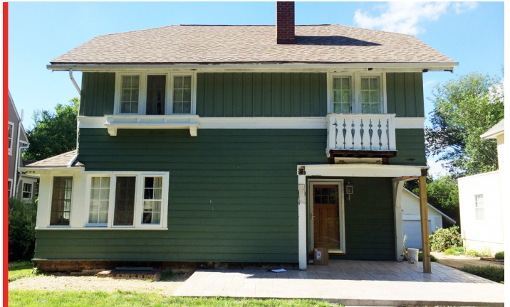
GREATHOUSE RESIDENCE BEFORE PORCH RENOVATION - PHOTO COURTESY OF BRIAN HAINES
