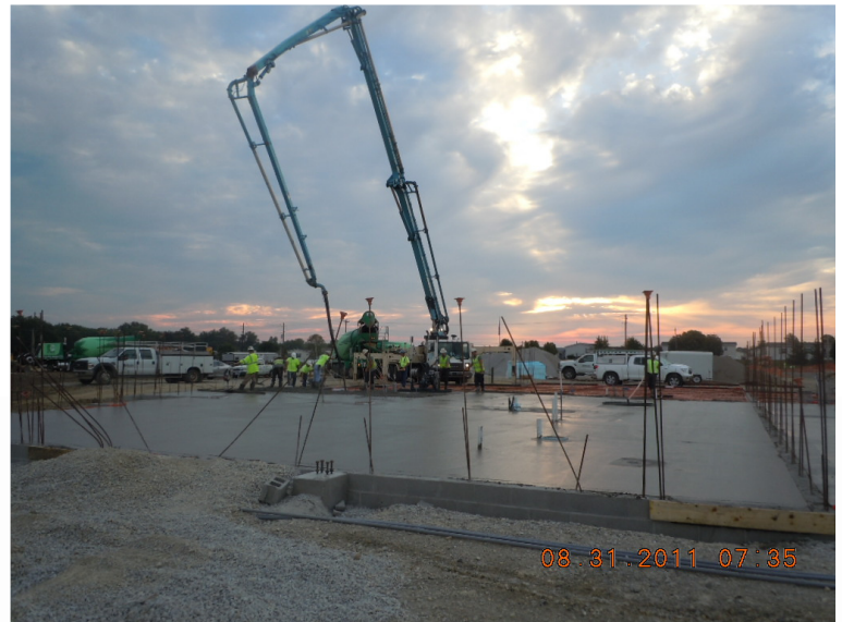
View of the Slab for the Administration Wing of the Public Works Facility after Early-Morning Pour —Photo Courtesy of Chris Godfrey
