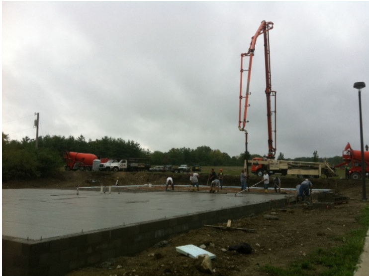
Slab Poured for 8,000 sqft Office Space at The Exchange on 741— Photo Courtesy of Joe Earley
