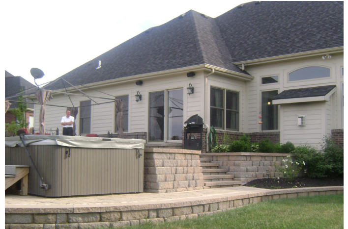
Existing Patio Space at Kalp Residence
