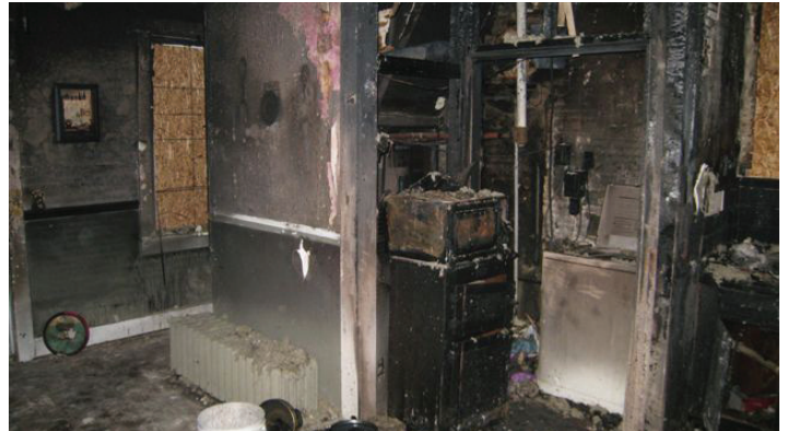
Wasmuth Kitchen/Utility Area After Fire Damage — Photo Courtesy of Adam Rose
