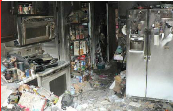
CURTIS RESIDENCE KITCHEN AFTER FIRE LOSS - PHOTO COURTESY OF ERIE INSURANCE
