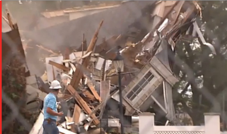
OTC SUPERINTENDENT, JAMES SKIPPER OVERSEES DEMOLITION OF FORMER L'AUBERGE BUILDING -PHOTO COURTESY OF DAYTON DAILY NEWS
