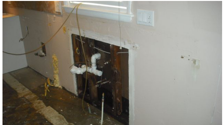
Kitchen in Stempson Residence Post Demolition
