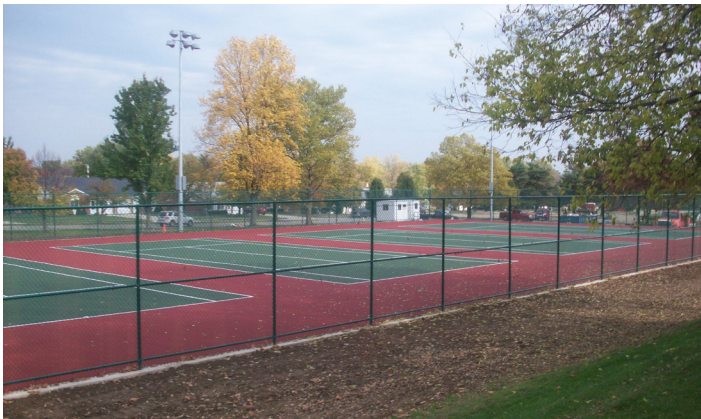
New Tennis Court Installed at Ernst Park
