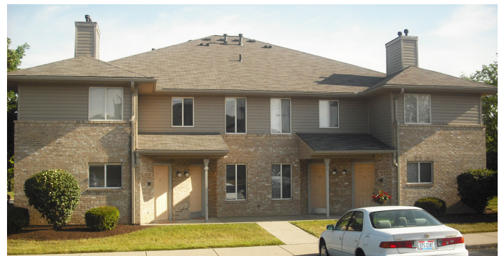
(After) Front Elevation of Mill Pond Unit with Clay Siding.
