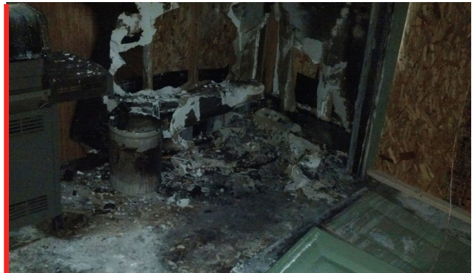
FIRE LOSS IN GARAGE AT KORTY RESIDENCE -PHOTO COURTESY OF MICHAEL JASKOLKA
