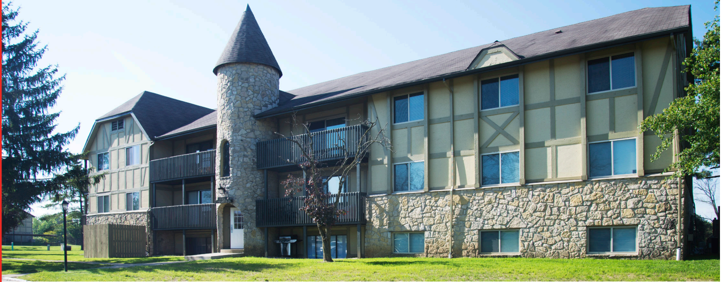
PHOTO OF RESTORED BUILDING AT STONEBRIDGE APARTMENT COMPLEX
