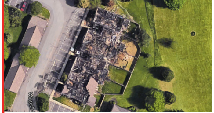
AERIAL PHOTO OF DAMAGED APARTMENT BUILDING AT FAIRWAY LAKES -PHOTO COURTESY OF GOOGLE EARTH
