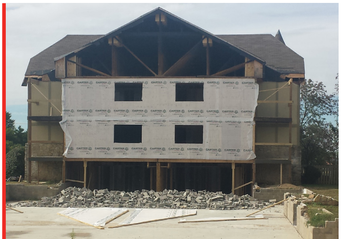
PROGRESS PHOTO OF WESTERN ELEVATION
