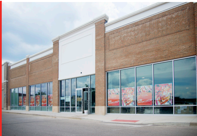
PROGRESS PHOTO OF ULTA BEAUTY (BEFORE SIGN INSTALL) -PHOTO COURTESY OF CAROLINE MORGAN
