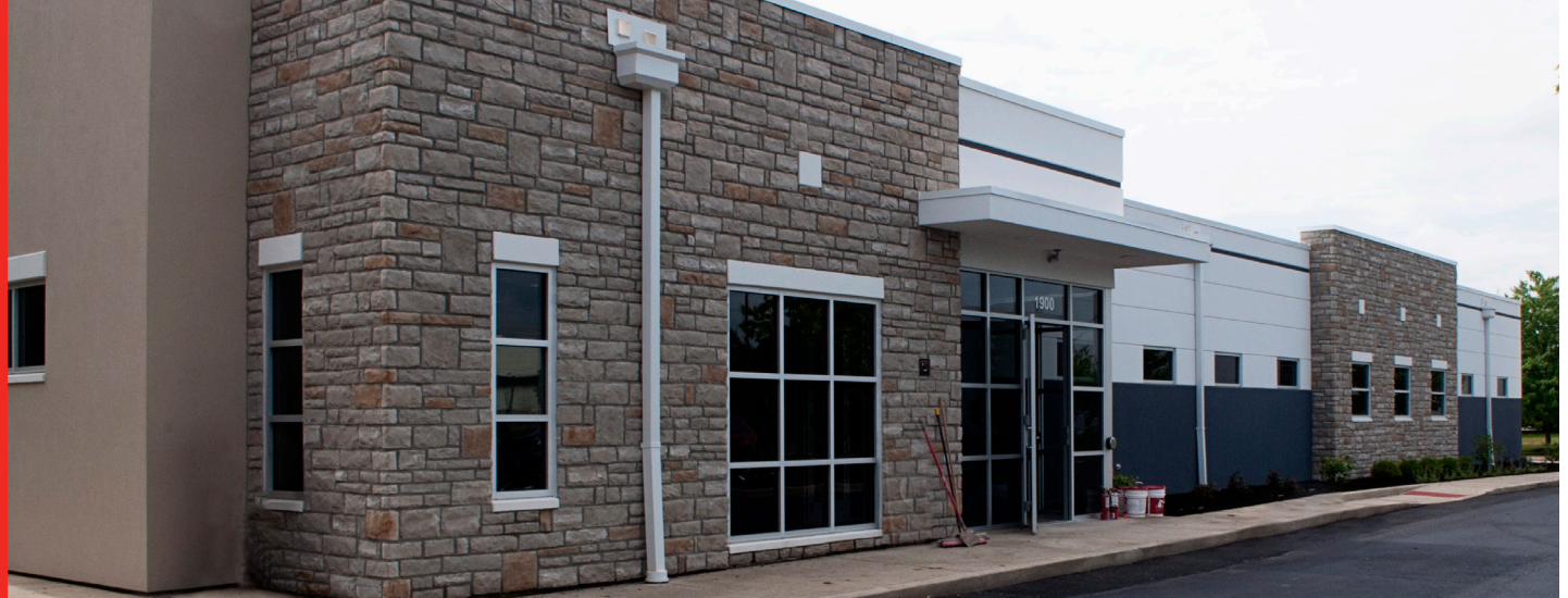
FRONT ELEVATION OF PriMED PATTERSON II LOCATED AT 1900 COMPOSITE DRIVE IN KETTERING - PHOTO COURTESY OF CAROLINE MORGAN
