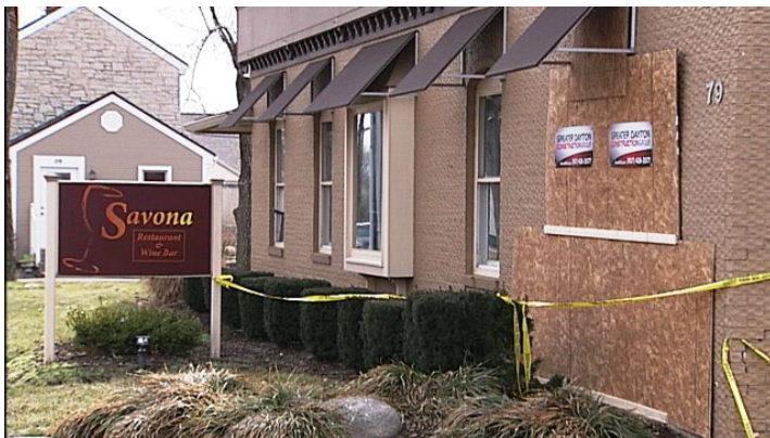
GDCG's Temporary Repairs to Savona Restaurant
