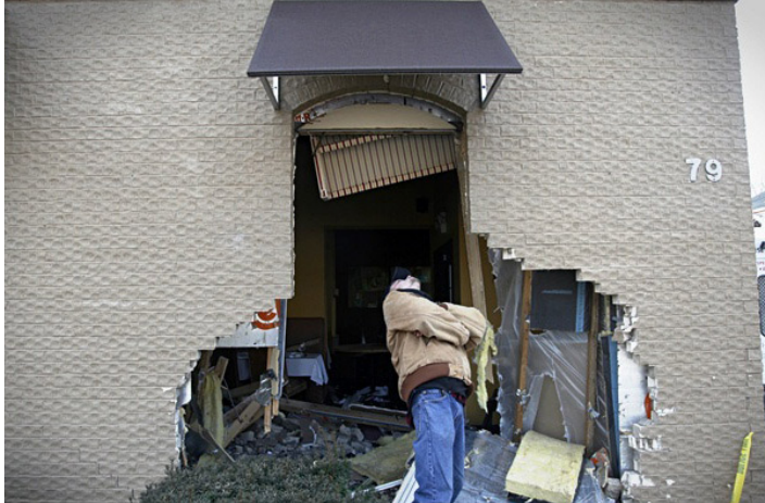
GDCG's Cody Treon Inspects the Vehicle Impact Damage to Savona Restaurant
