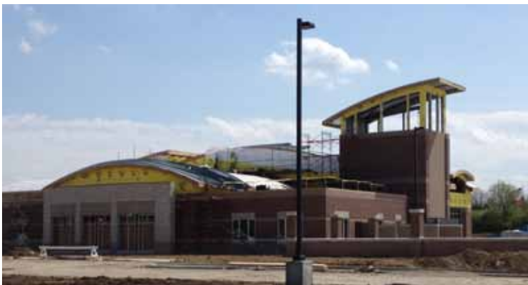
Miami Township Fire Station – 11 Months Into Production – Photo Courtesy of Chris Godfrey
