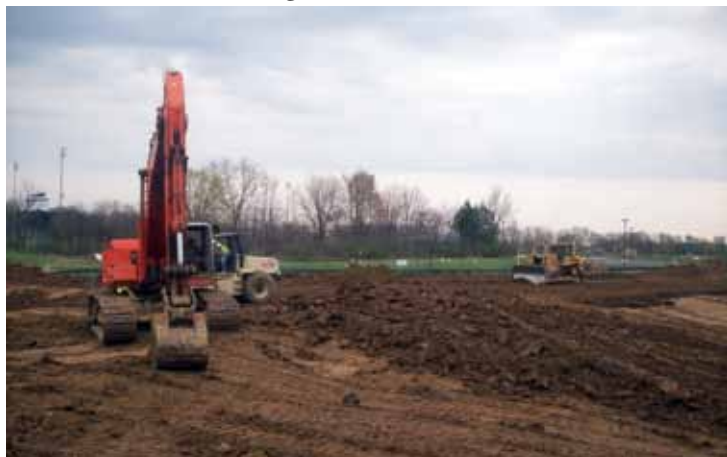
Site Work Begins at Olentangy Crossing
