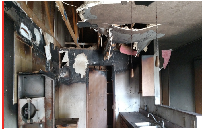
PHOTO OF WILLIAMS KITCHEN AFTER FIRE LOSS -PHOTO COURTESY OF DAVE WILSON
