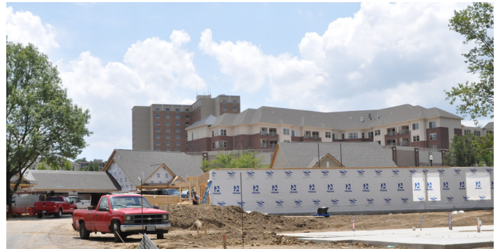
Grand Cottages Under Construction at Bethany Village – Photo Courtesy of Caroline Morgan
