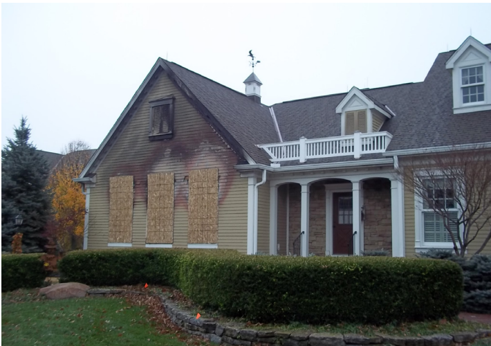
Fire Damage to Garage of Swormstedt Residence (Final Picture to be Included in July Edition)
