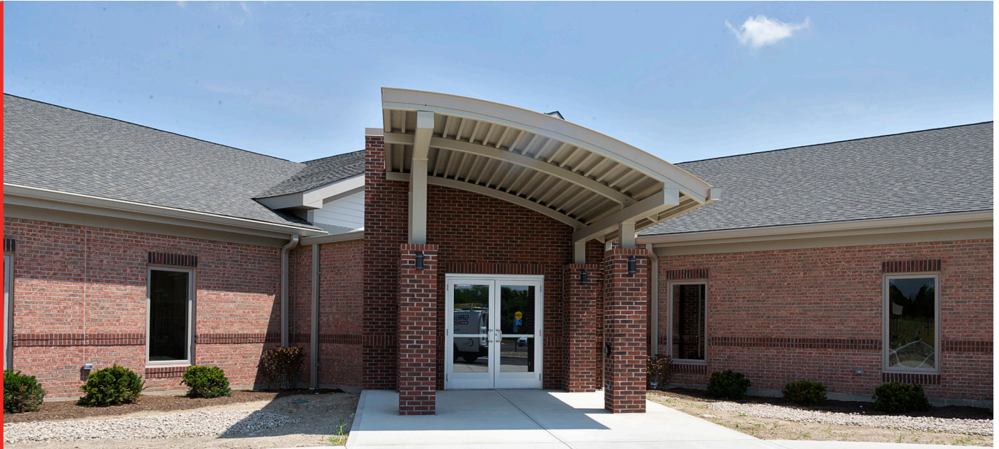
FRONT ELEVATION OF PROJECT C.U.R.E.'S NEW TREATMENT FACILITY IN MORAINE
