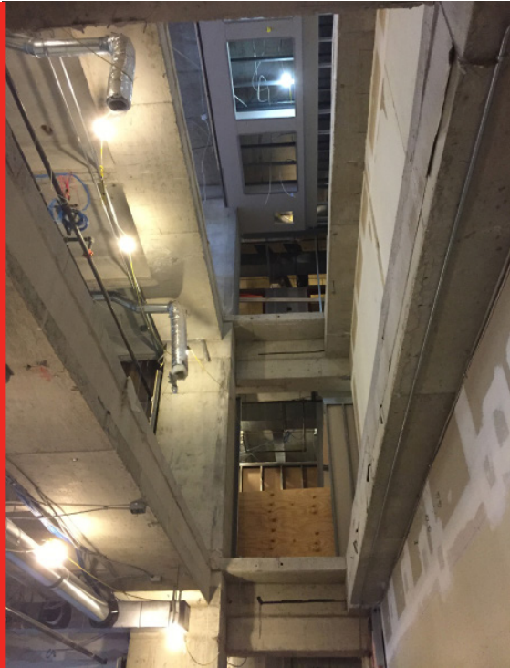
PROGRESS PHOTO OF SLAB DEMOLITION FOR STAIRCASE AT DINSMORE & SHOHL - PHOTO COURTESY OF GENO TARTELL
