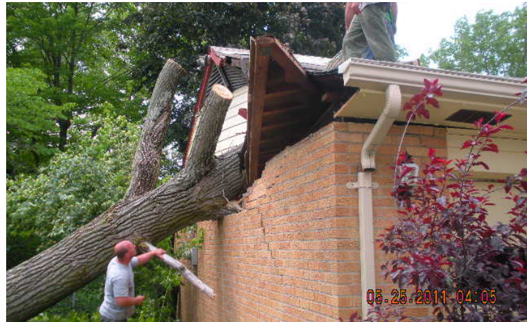
Example of High Winds Damage to the Miles Residence in Dayton— Photo courtesy of Tom Carney
