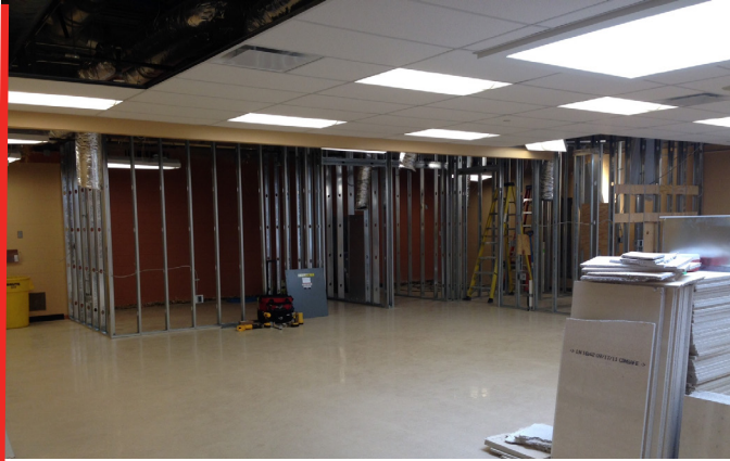
IN PROGRESS PHOTO OF CLASSROOM FRAMING -PHOTO COURTESY OF JOHN REAGAN
