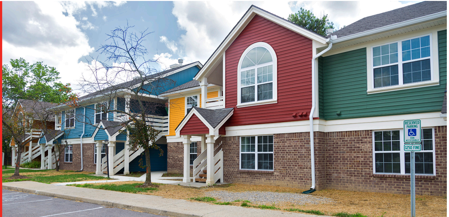
FRONT ELEVATION OF MAD RIVER APARTMENTS AFTER RESTORATION EFFORTS
