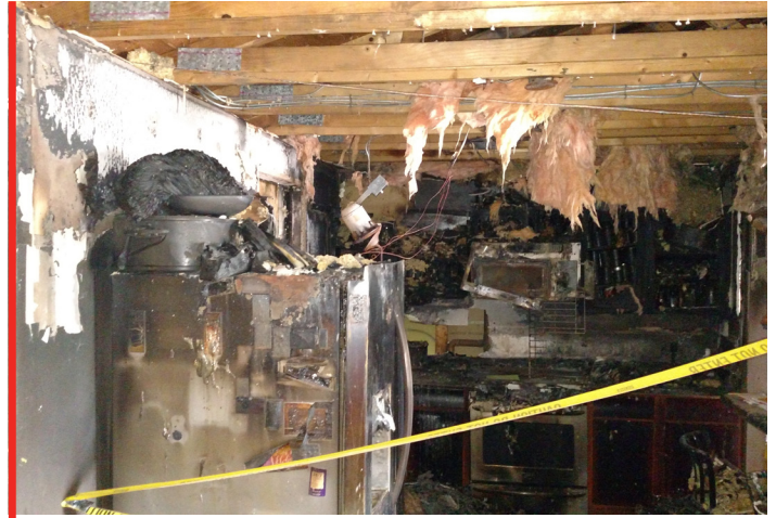
KITCHEN IN MURRAY RESIDENCE AFTER FIRE LOSS -PHOTO COURTESY OF MICHAEL JASKOLKA
