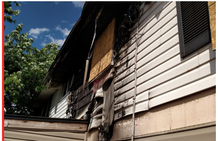
EXTERIOR DAMAGE AT MURRAY RESIDENCE AFTER FIRE LOSS -PHOTO COURTESY OF MICHAEL JASKOLKA
