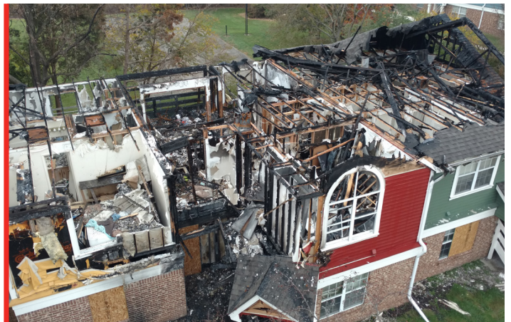
AERIAL PHOTO OF MAD RIVER APARTMENTS AFTER FIRE LOSS
