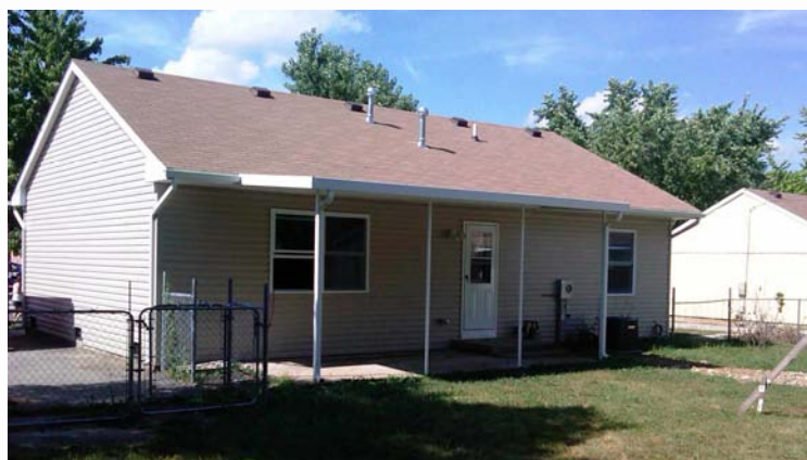
Burke Residence “After” Picture Following Restoration Efforts— Photo Courtesy of Earl Wyatt
