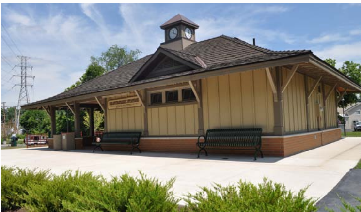
Beavercreek Station Restroom Facility— Photo Courtesy of Caroline Morgan
