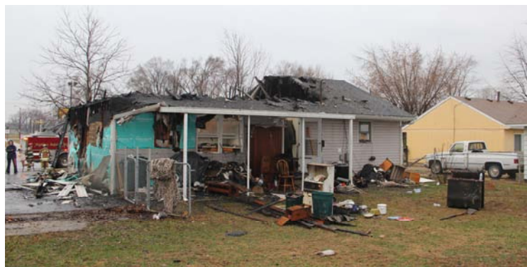
Burke Residence “Before” Picture Following Total Fire Loss— Photo Courtesy of Mike Jaskolka
