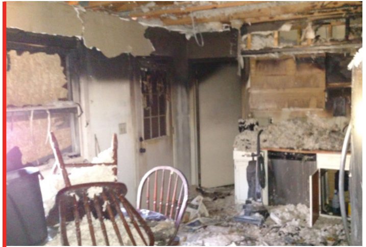
PHOTO OF KNOX KITCHEN AFTER FIRE LOSS
