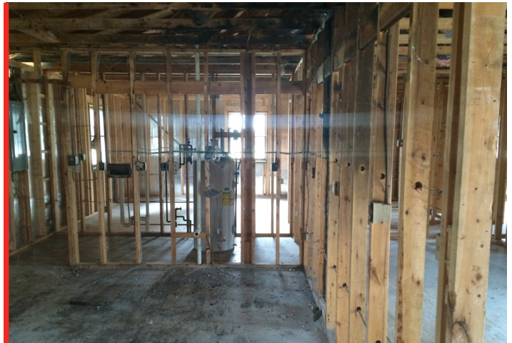
PROGRESS PHOTO OF KITCHEN DURING RESTORATION EFFORTS (BEFORE SPRAY SEAL)
