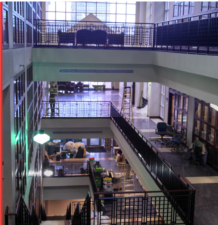
RESTORATION EFFORTS IN PROGRESS AT THE UNIVERSITY OF DAYTON LAW LIBRARY BUILDING
