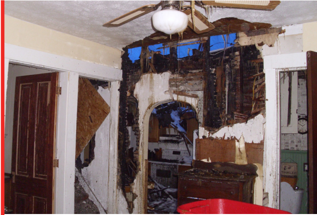
ELROD RESIDENCE FIRE DAMAGE -PHOTO COURTESY OF DAVID WILSON
