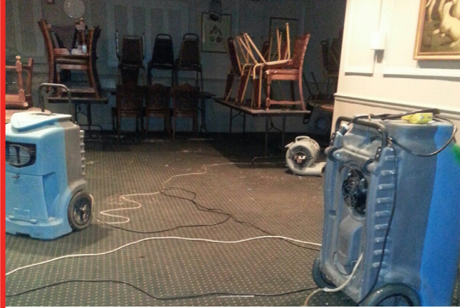
MOISTURE EXTRACTION UNITS WORK TO DRY OUT THE CARPET AT THE BARNSIDER RESTAURANT
