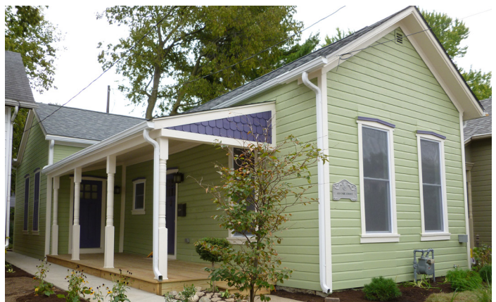
Front Elevation of 634 Oak St. After Renovations
