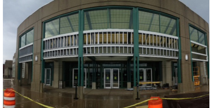
Progress Photo of Gate 3 Renovations at Ervin J. Nutter Center
