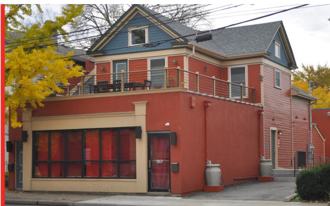
FRONT ELEVATION OF 1207/1209 WAYNE AVENUE AFTER RENOVATIONS
