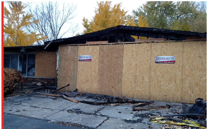
MATLOCK RESIDENCE AFTER BOARD-UP EFFORTS - PHOTO COURTESY OF DAVE WILSON
