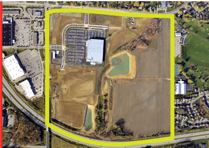
AERIAL PHOTO OF THE CORNERSTONE DEVELOPMENT AFTER SITE-PREPARATION EFFORTS AND CONSTRUCTION OF COSTCO BUILDING - PHOTO COURTESY OF OBERER LAND DEVELOPERS
