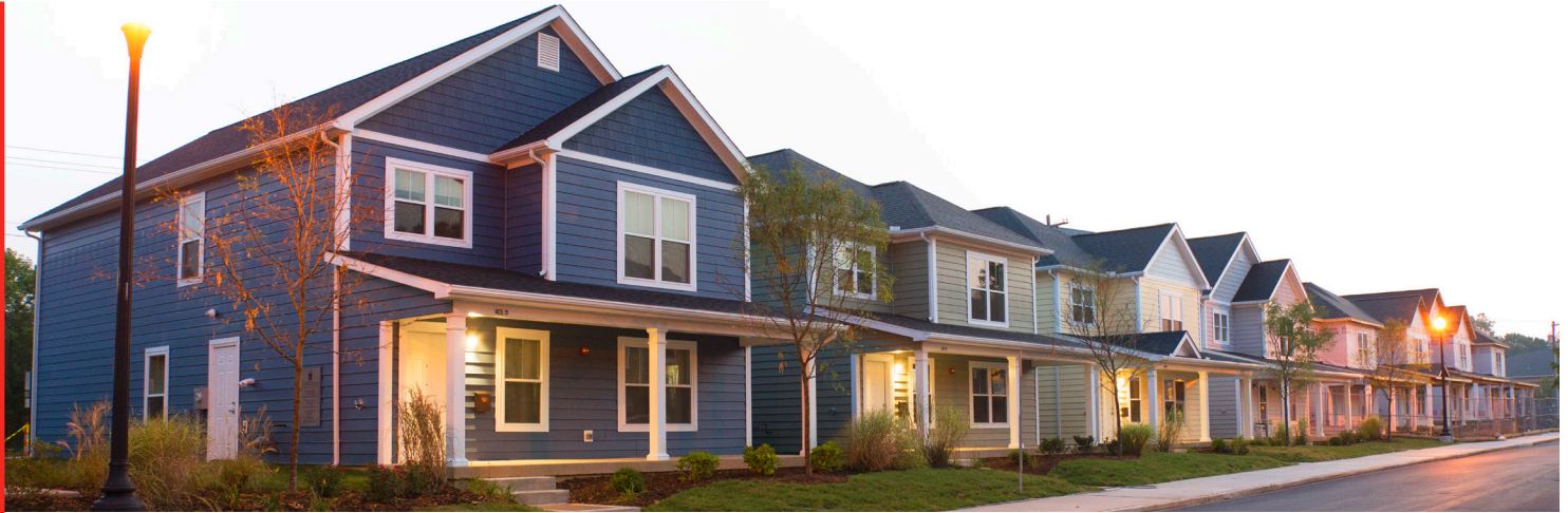
PROGRESS PHOTO OF NEW STUDENT HOUSING AT THE UNIVERSITY OF DAYTON (“I LOVE U.D.” HOUSE, FAR LEFT)
