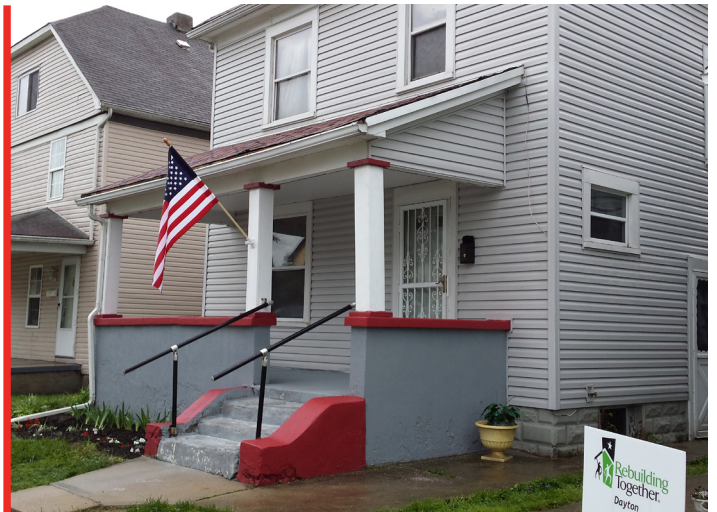
EXTERIOR OF ERMA COOPER'S HOME AFTER RENOVATION EFFORTS FROM REBUILDING TOGETHER'S VOLUNTEERS - PHOTO COURTESY OF JOHN POPELAR
