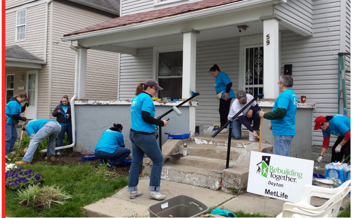
VOLUNTEERS HELP WITH RENOVATIONS DURING NATIONAL REBUILDING DAY 2015 - PHOTO COURTESY OF JOHN POPELAR
