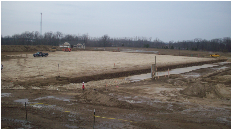
Kohl's Building Pad--Photo courtesy of Tony Quinter
