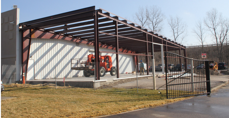
GDCG Building Addition Progress--Photo courtesy of Tom Carney
